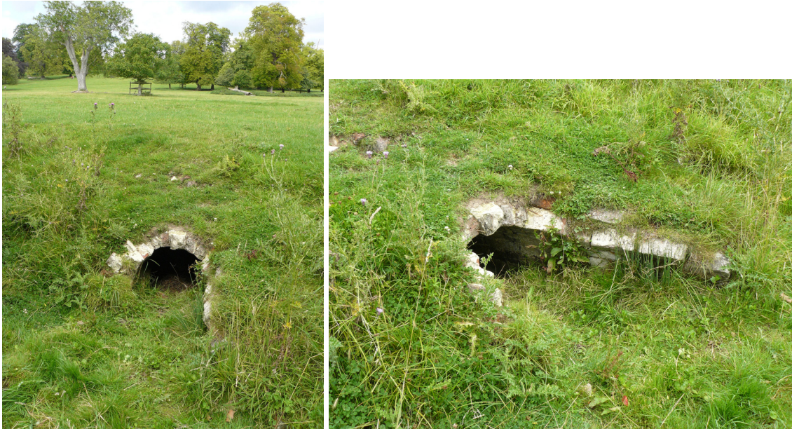
Conduit outfall photographs.
